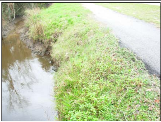
SOUTH END (FROM EAST)
